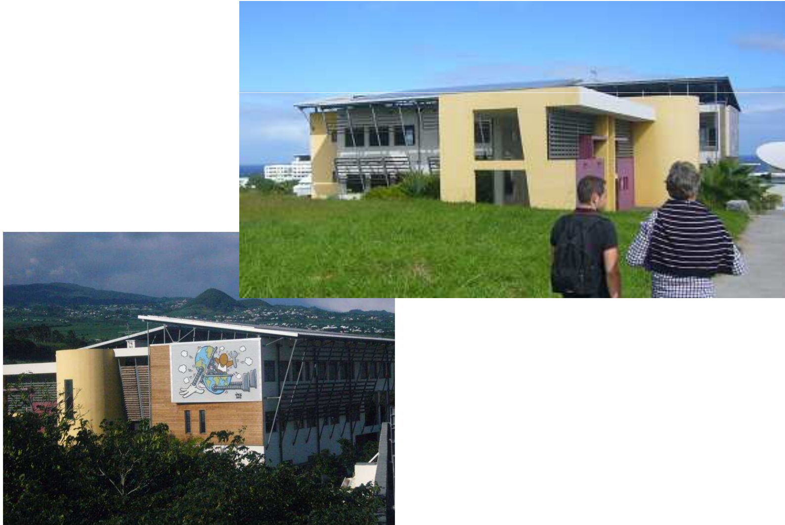
JUMELAGE Eco - Construction
