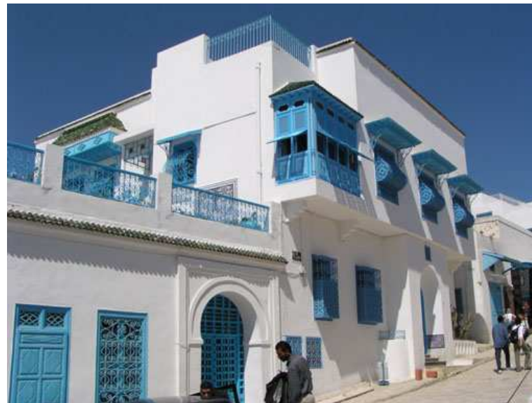
JUMELAGE Eco - Construction
